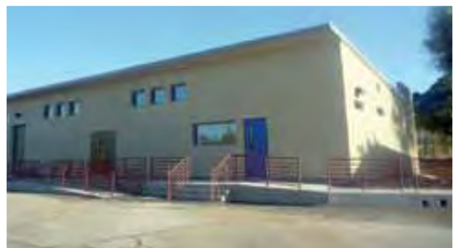
New building is ready to serve! A walkway canopy will be added January 2012 for added comfort for recipients.
