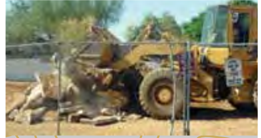
Bye-Bye Old Storage Shed: The construction begins July 2 nd .
